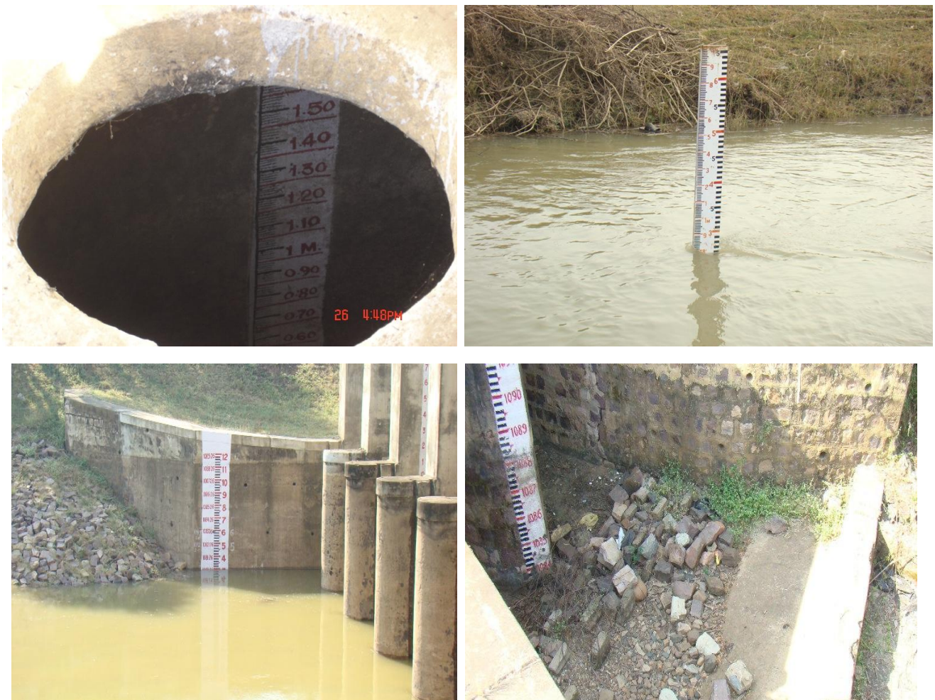
Photo 9 Sump Well, Scale on the Distributary, Scale at the Cross Regulator and Scale at Gate
